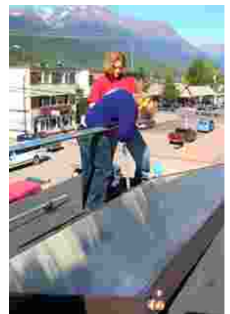
Installing One Sky's solar hot water heater
