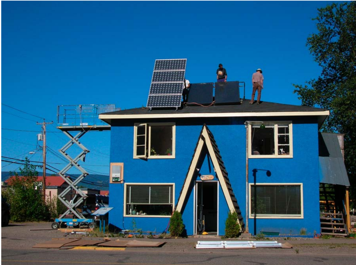
One Sky office during PV net-meter installation, August 2006
