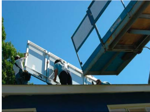
Installing PV system on One Sky roof.
