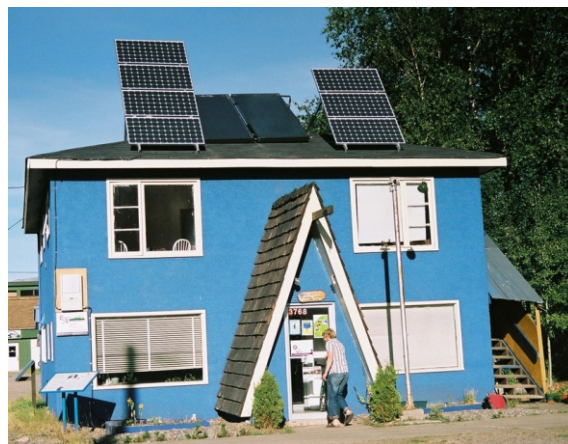
One Sky's Smithers office demonstrating net-metered PV system and solar hot water heater.
