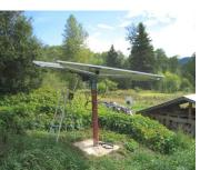
once their energy demands started to grow they added two more solar panels in 1996, and then recently, another eight 110-watt panels mounted on a Wattsun tracker© (cost \$3000). The tracker maximizes sun exposure as it moves with the sun throughout the day thereby maximizing power generation. The system is located about 160 feet from the battery bank, which in turn ranges from 8 to50 feet from the electrical load. Efficiencies are lost with distances.
